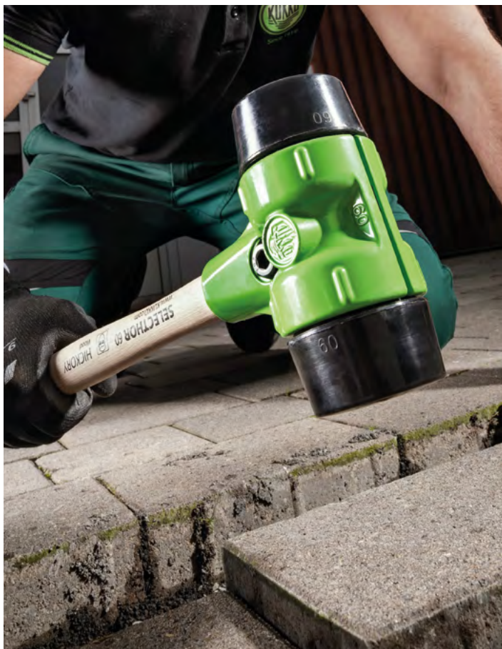
Use of a Schonhammer Selector when laying paving stones
